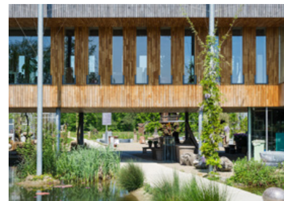
The old company building was taken down and then rebuilt in the new location.
